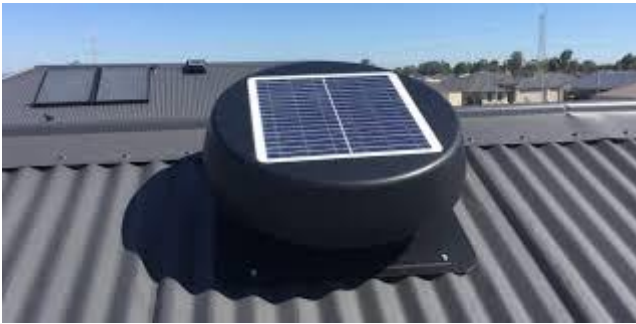
Photo 1 Solar power ventilation
