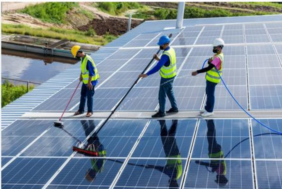
Figure 11: Solar PV maintenance. Source: https://rkwindmast.com/c/can-you-power-wash-solar-panels.html
